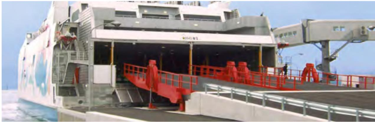
Tailor made MacGregor linkspans for the rampless catamarans are installed in Hakodate and Aomori in Japan. The hydraulically operated linkspans allow quick operation and smooth vehicle transfer across the full breadth of the catamarans.
