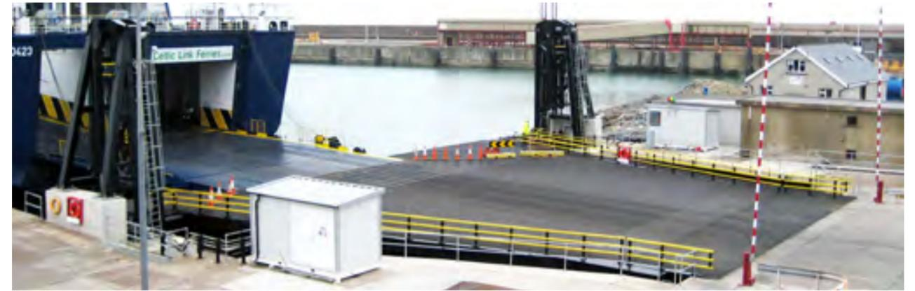
The linkspan is large for an articulated ramp. The seaward ramp interface is 34m wide and the ramp is 20m wide at the shoreside end. It is 30m long in order to cater for the local tidal conditions as well as most ships' thresholds.
