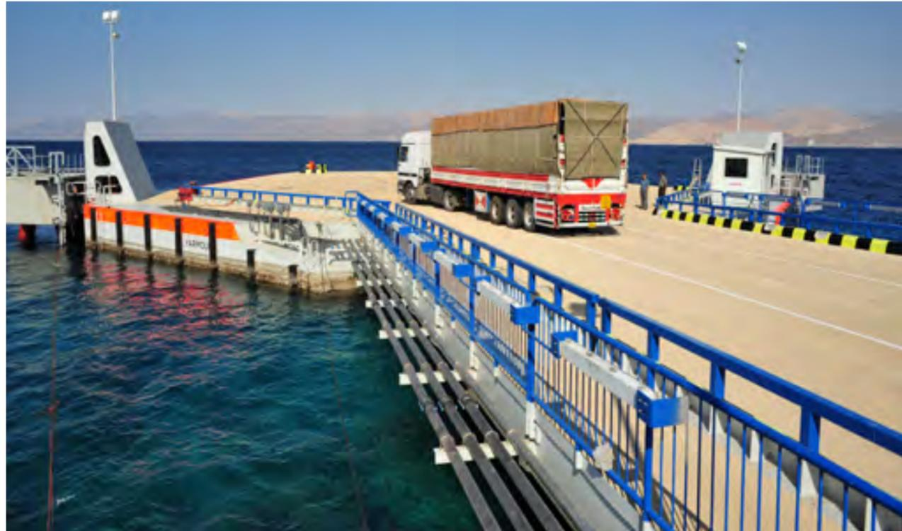
The large hexagonal floating pontoon linkspan was a supply chain challenge. A slipway was constructed at the production site in Croatia to ensure the equipment's safe launch. It was towed across the Mediterranean, through the Suez Canal, around Sinai, to its final destination in Aqaba Ports, Jordan.
