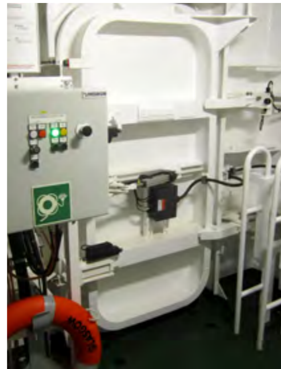
Electrically-driven shell door.
