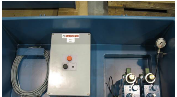
Wireless control unit
