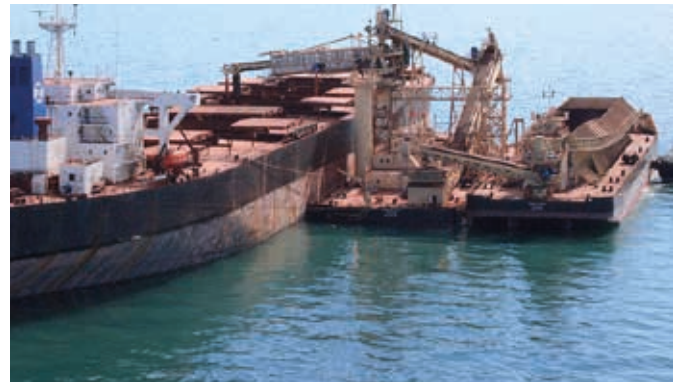
Transfer terminal systems
