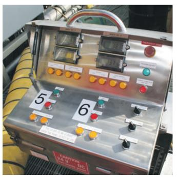
Local control console for operating MacGregor RamWinches on board the *Blind Faith semi*.
