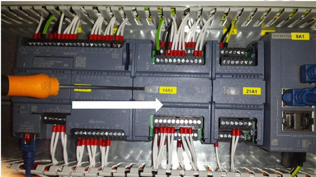
Figure 1: Open the bus connector
