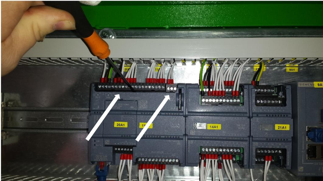
Figure 2: Disconnect upper terminal strip
